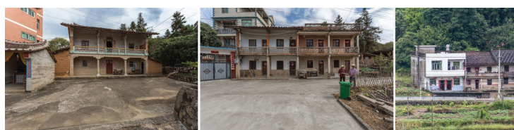
Figure 4: Evidence of "village hollowing." Vacant dwellings in sound condition. Source: Photos by Semprebon (Sept 2018).
