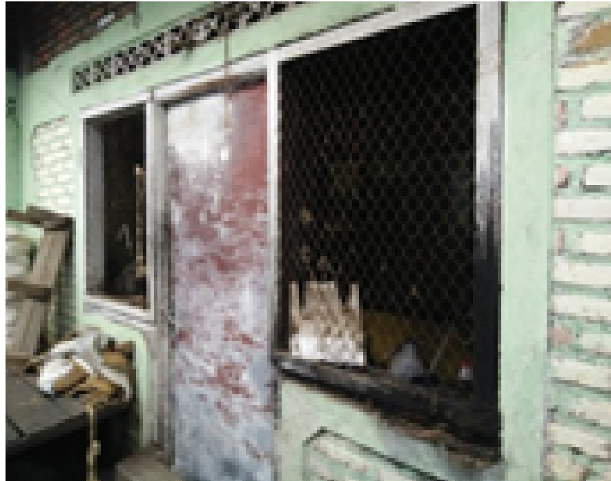
Figure 1: Picture of buildings condition. (Source: Author's collection.)
