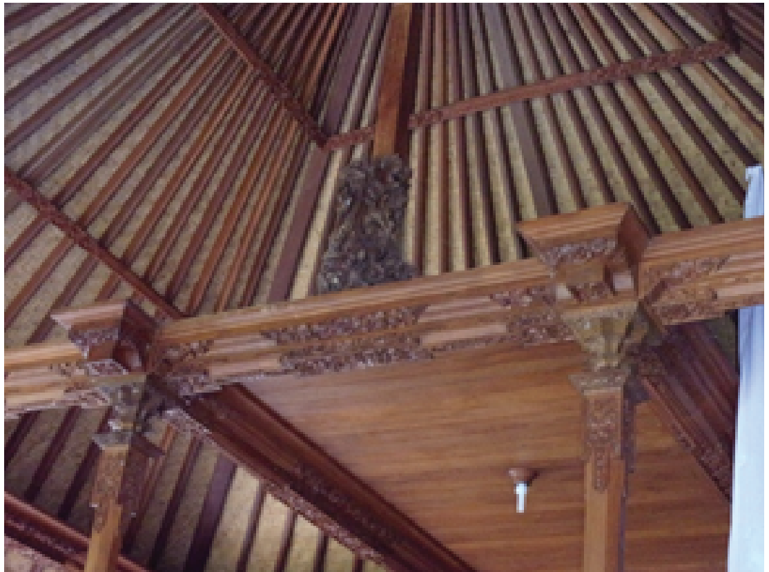
Figure 3: Roof construction of bale – Jro Kuta, Denpasar.
