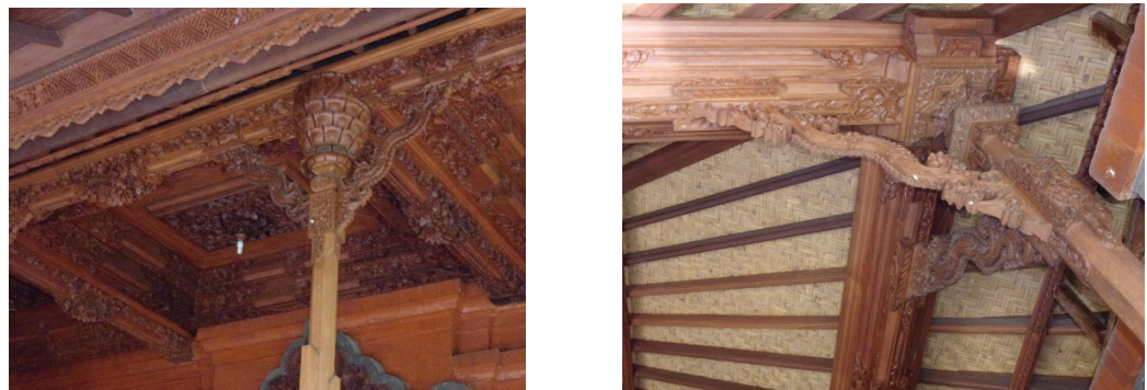
Figure 5: Poles and beams joint applied in bale - Jro Kuta, Denpasar.
