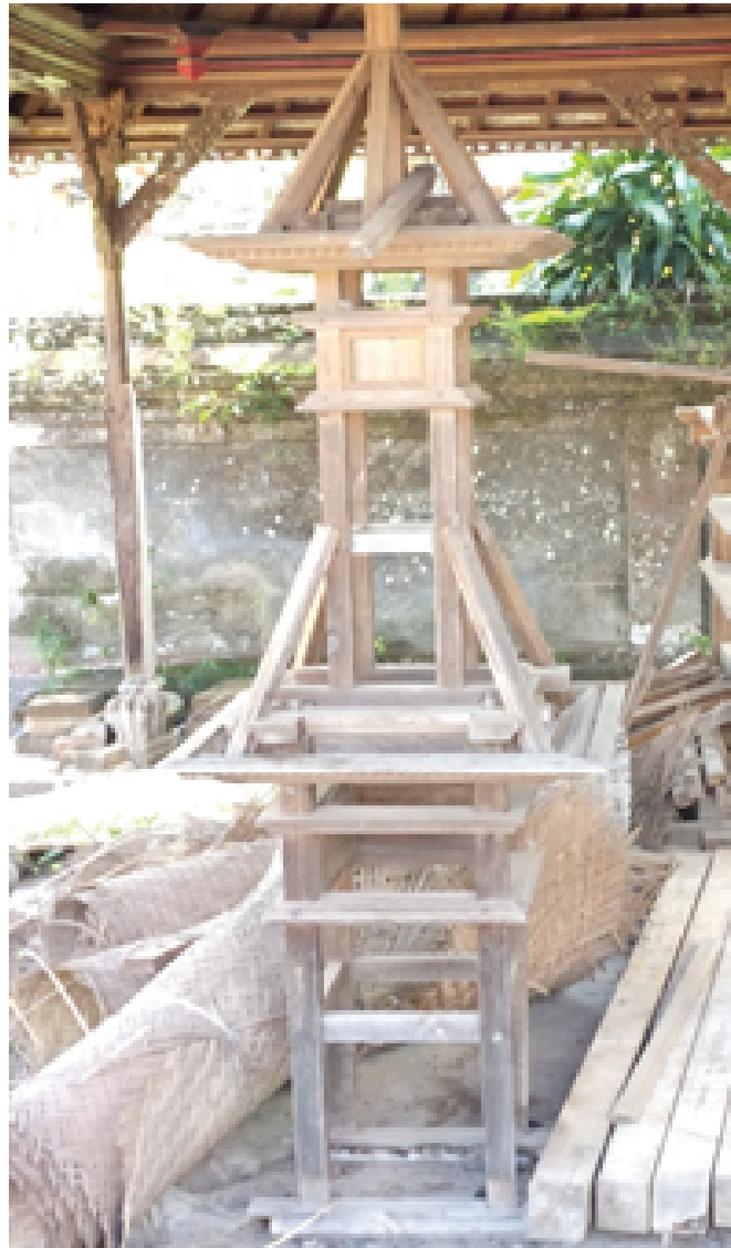
Figure 2: Roof construction of shrine – Pura Taman Sari, Klungkung.
