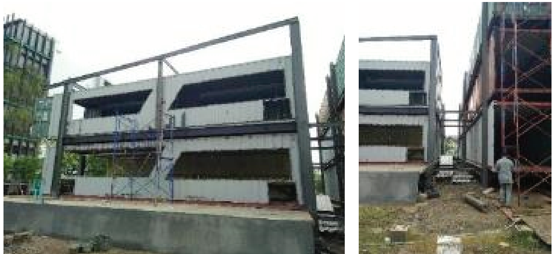
Figure 7: implementation of structure system at construction site.
