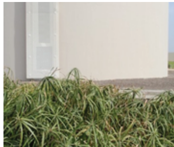
Figure 8: The constructed wetland for natural water treatment installed behind the EcoHaus.
