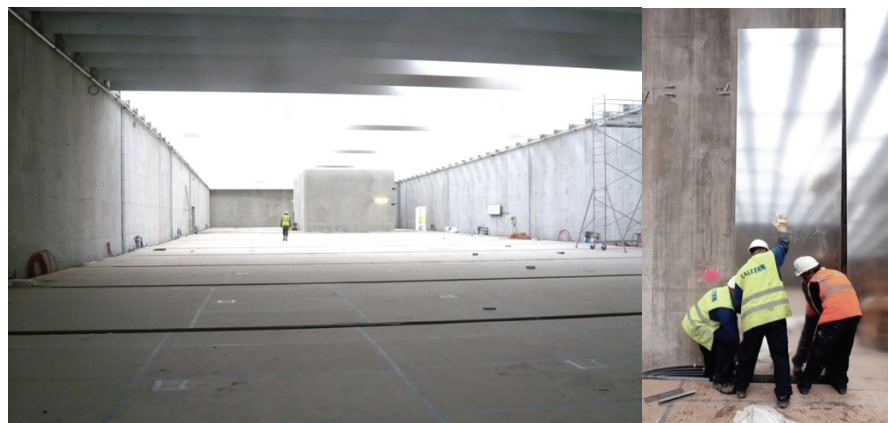
Figure 3: Exhibition gallery of the Louvre-Lens Museum under construction.
