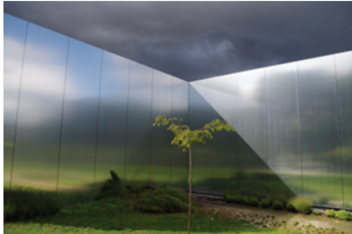
Figure 6: Louvre-Lens Museum: Grey sky and reflection of clear sky on the aluminium walls.
