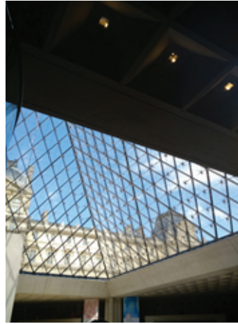
Figure 6: View from the inside to the outside (Photographed on site, 2015).
