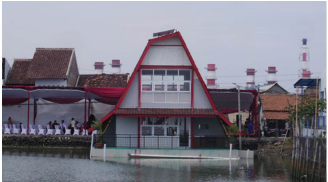
Figure 2: Biofilter installed on side the main Tambak Lorok library floating structure.
