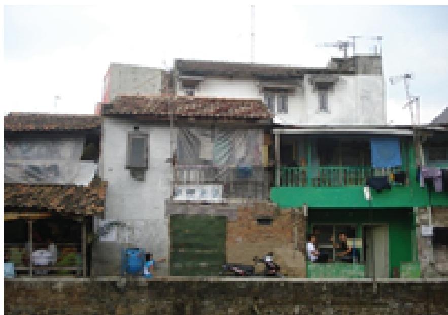
Figure 9: The building quality in Cidurian riverbank settlement.
