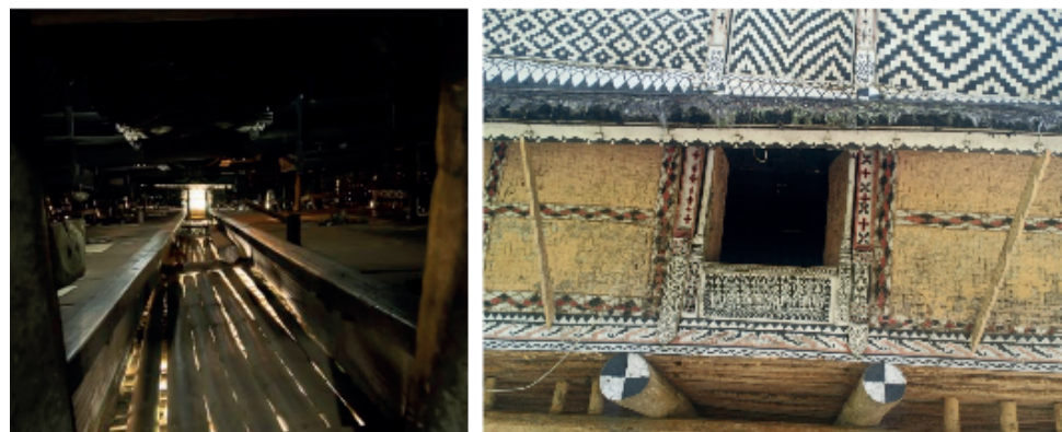
Figure 3: Interior of the front area of the house. Source: Personal documentation.
