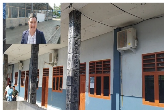
Figure 3: All student rooms have been facilitated with air conditioning.
