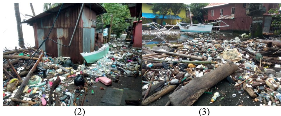
Figure 2: Settlement Condition in Coastal Areas of Mallusetasi Sub-District.
