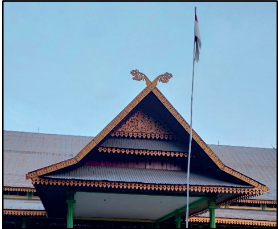
Figure 1: Selembayung on a Traditional House.
