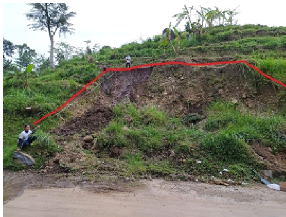
Figure 1: Landslide on Pacet-Trawas Road Corridor, Pacet District (Coordinate 6703980 mE, 9151868 mN) .
