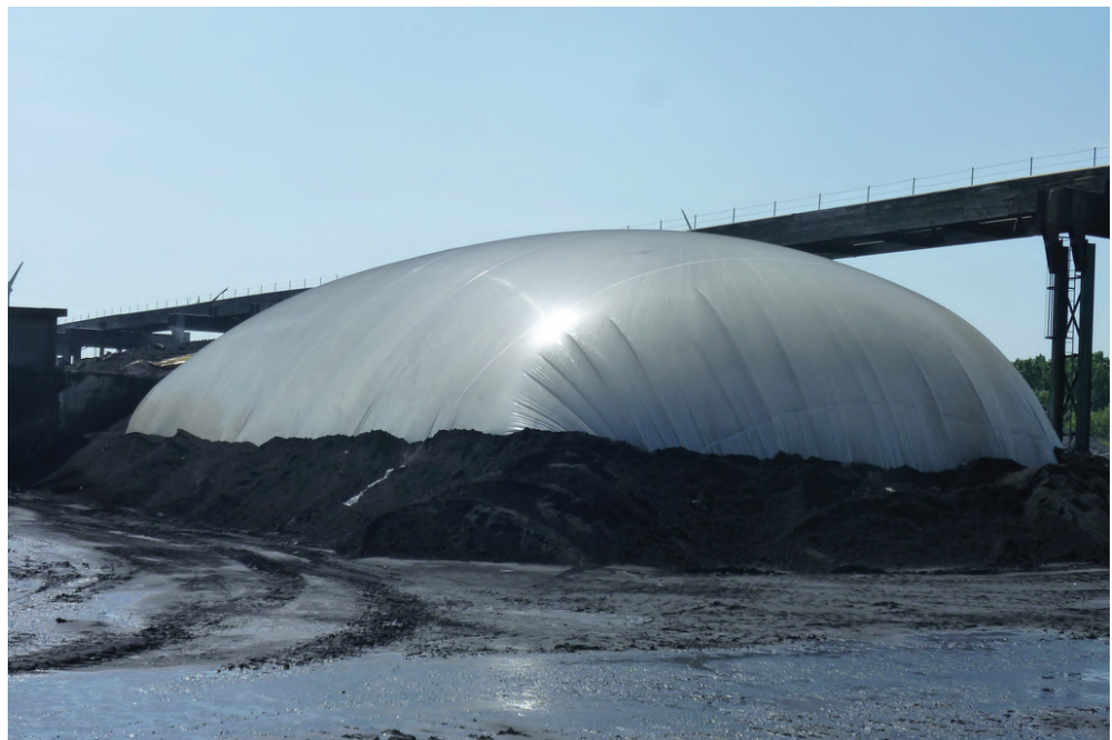
Figure 4: Stationary furnace of the open type with a system for collecting reaction gases at the plant ESK-SiC in Netherlands.
