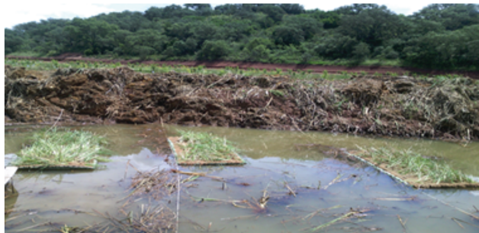
Figure 2: Field Installation of floating beds.
