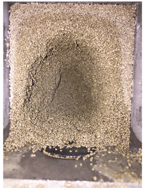
Internal of pit
