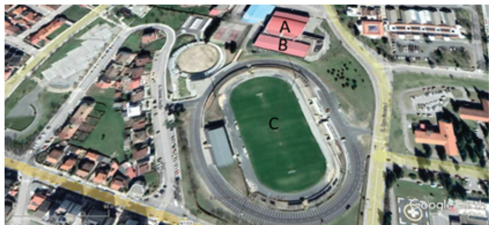
Figure 1: Plan of the Bragança municipal sports center: indoor football court (A) pools (B) and football stadium (C) (source: Google Earth).
