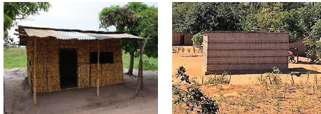
Figure 3: Construction with covering straw walls and roofing of metal sheet, in the central and southern area of Mozambique respectively.
