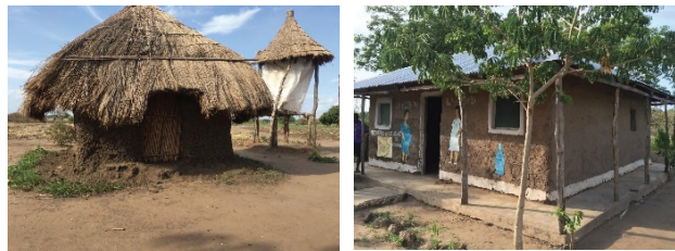
Figure 1: Construction of covering land and cover in the stem of the right and cover in metallic sheet in the construction of the Left, in the Wine Community.
