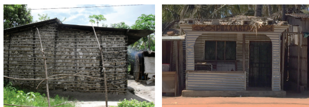
Figure 4: Construction with walls consisting of stones in the area of Dondo, on the left and construction with walls consisting of sheet metal cladding in the southern area of Mozambique, on the right.
