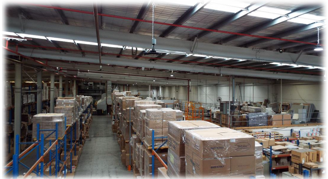
Figure 4: Energy efficient, wirelessly controlled, industrial lights (image courtesy of ESIC Lighting).
