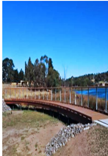
Figure 1: existing bridge (image courtesy of City of Greater Geelong).
