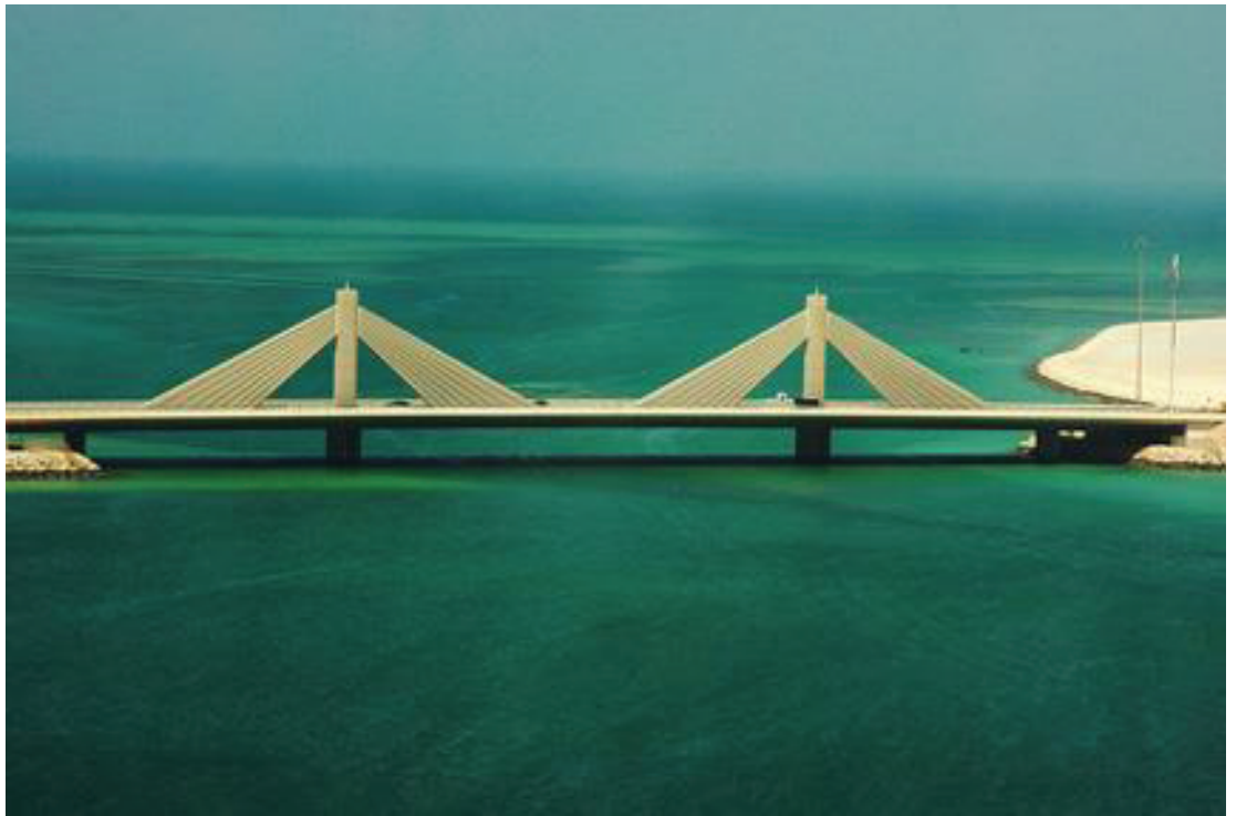
Figure 1: Triangular white columns of Shaikh Isa bin Salman Causeway (Haji Hassan ReadyMix 2012).
