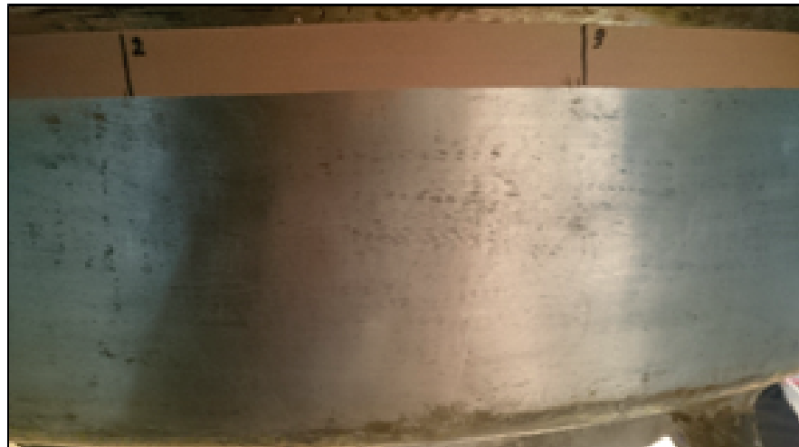
Figure 3: Fragment of the welding node of the cold collector of the sample of the steam generator with the welded joint.
