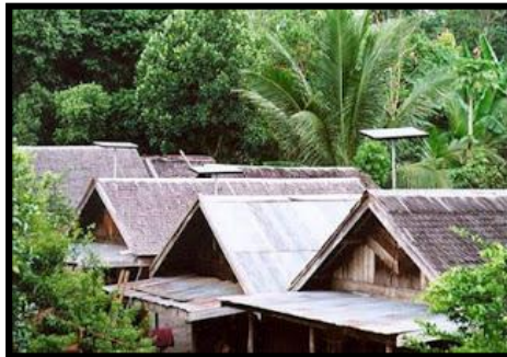
Fig. 1. The installation of solar cell.
